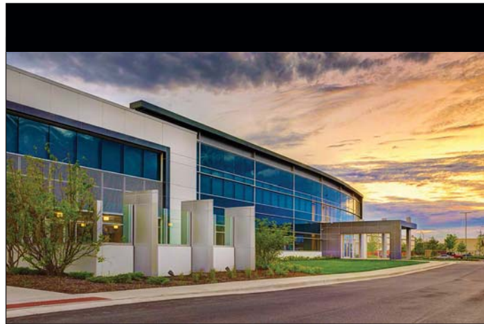
The design/build construction of the new 165,230 square foot LEED-Gold Regional Headquarters for Golden State Foods, featuring a sophisticated CO 2 cascade refrigeration system, was recently completed by McShane Construction and Ware Malcomb in McCook, Illinois.
